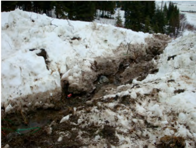
February: Drainage ditches for water pumped from peoples basements
